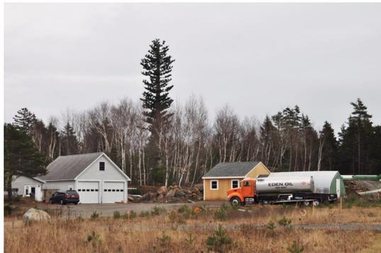
*Figure 23: Survey Image, Cell Tower Disguised as Monopine*
