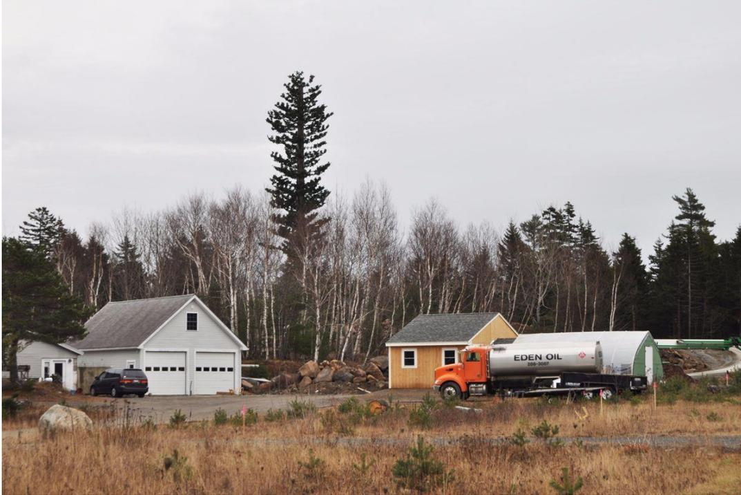
*Figure 1: Disguised as White Pine Cell Tower (Broom, Dick, 2015)*
