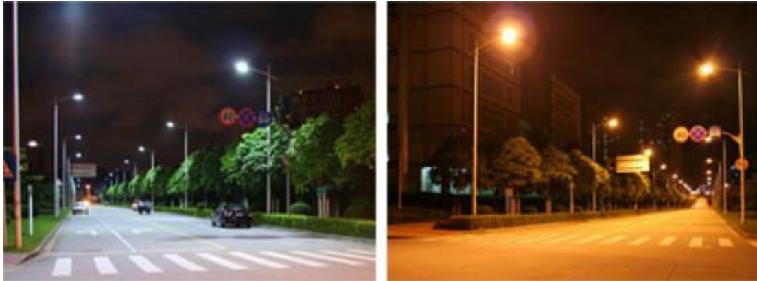
Figure 3: On the left is a road lit by new LED Street Lights, on the right is the same road using old high pressure sodium lights. The new lights clearly increase visibility while using much less energy [13].
