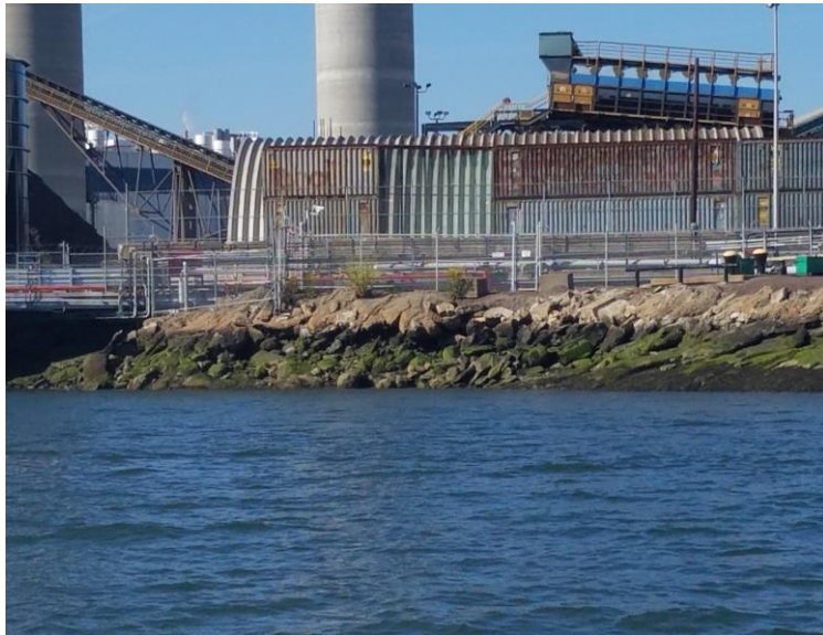
Figure 9: Riprap located at Prolerized
