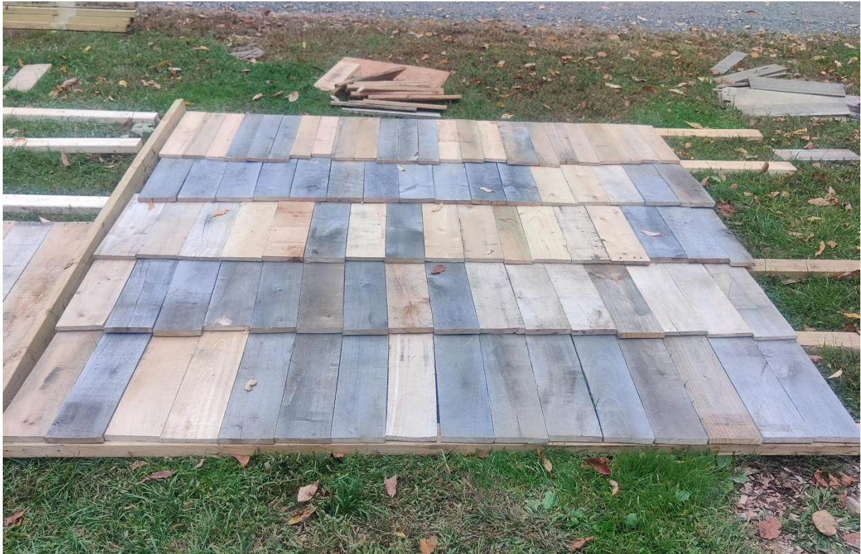
Figure 10: A wall using the pallet wood.
