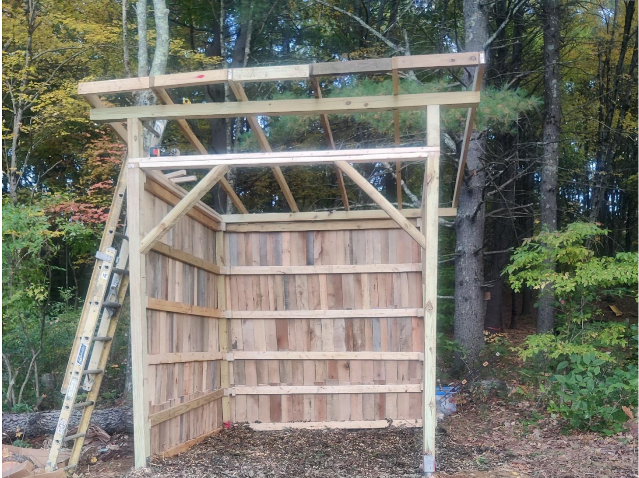
Figure 14: the Lodge with both walls installed, and the rafters installed.
