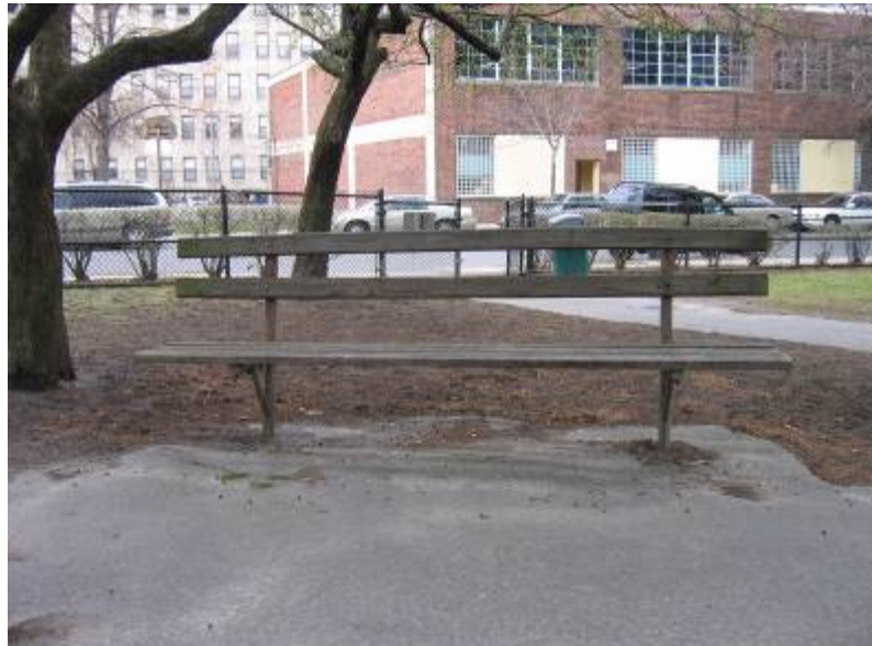
Figure 2 - Bench in Violation due to lack of armrests
