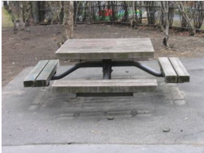
Figure 3 - Non-accessible picnic table due to lack of required space for wheelchairs
