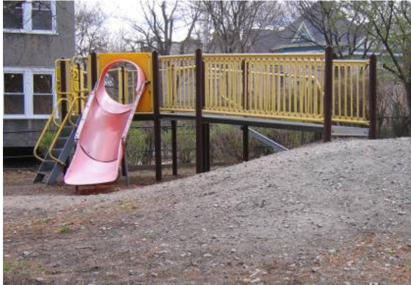
Figure 5 - Composite Climbing Structure
