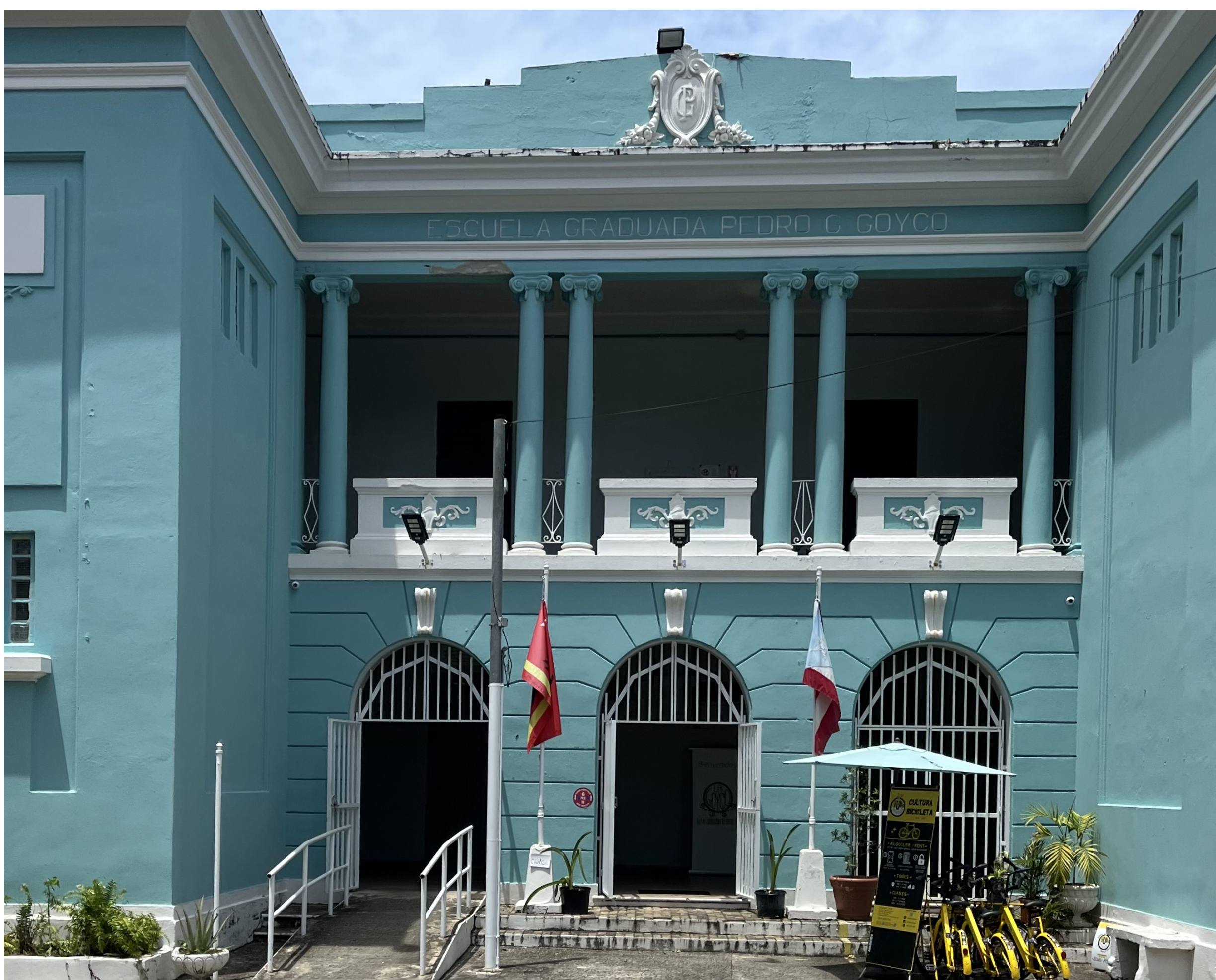
Figure above shows the school building that La Goyco repurposed.
