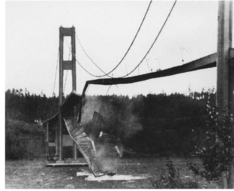
Figure 5: The collapse of the Tacoma Narrows Bridge (Matsumoto, Shirato, Yagi, Shijo, Fguchi, & Tamaki, 2003)
