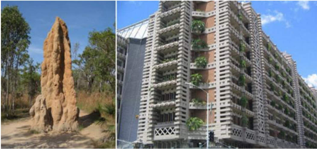
The EastGate Centre in Zimbabwe (right), inspired by termite mounds (left) for natural ventilation and temperature control. (Nkandu & Alibaba, 2018; Singh & Nayyar, 2015).
