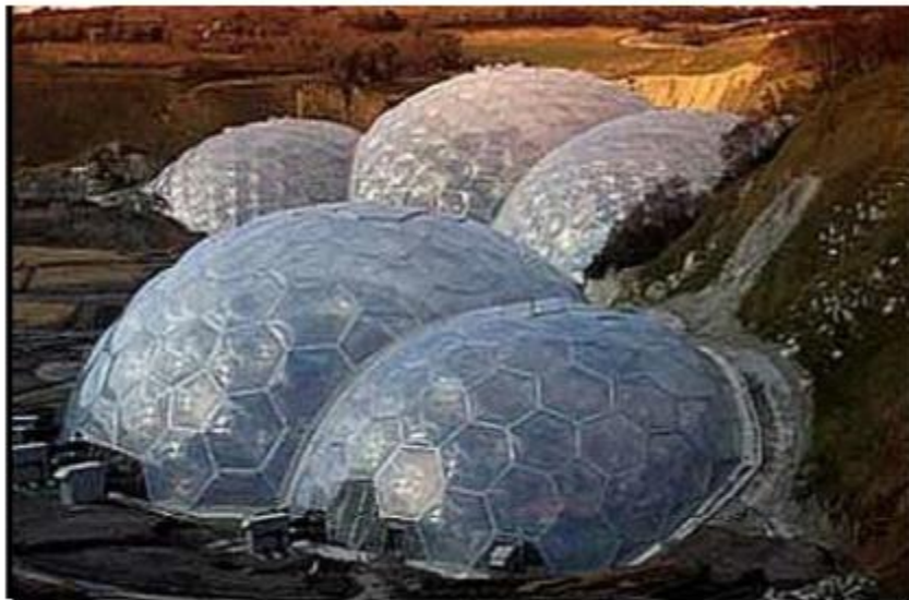
Geodesic domes of the Eden Project in Cornwall, England, inspired by “soap bubbles and pollen grains”, that maximize surface area versus weight (Singh & Nayyar, 2015).
