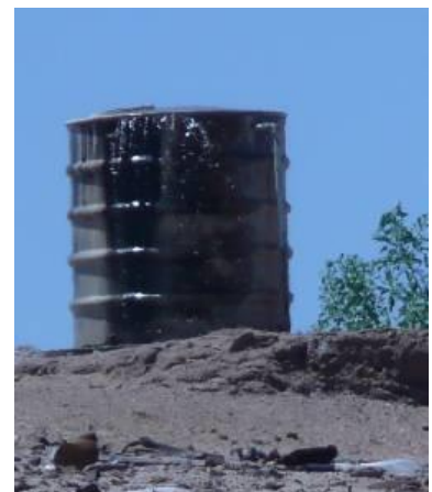
Figure 34: Overflowing water tank
