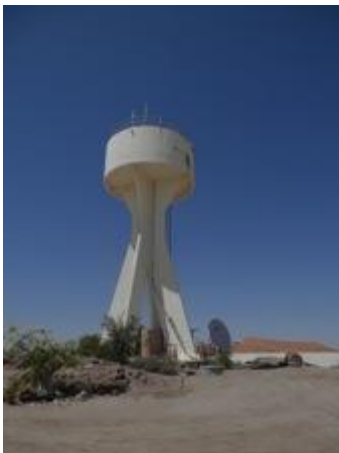
Figure 7: GRTC Water Tower
