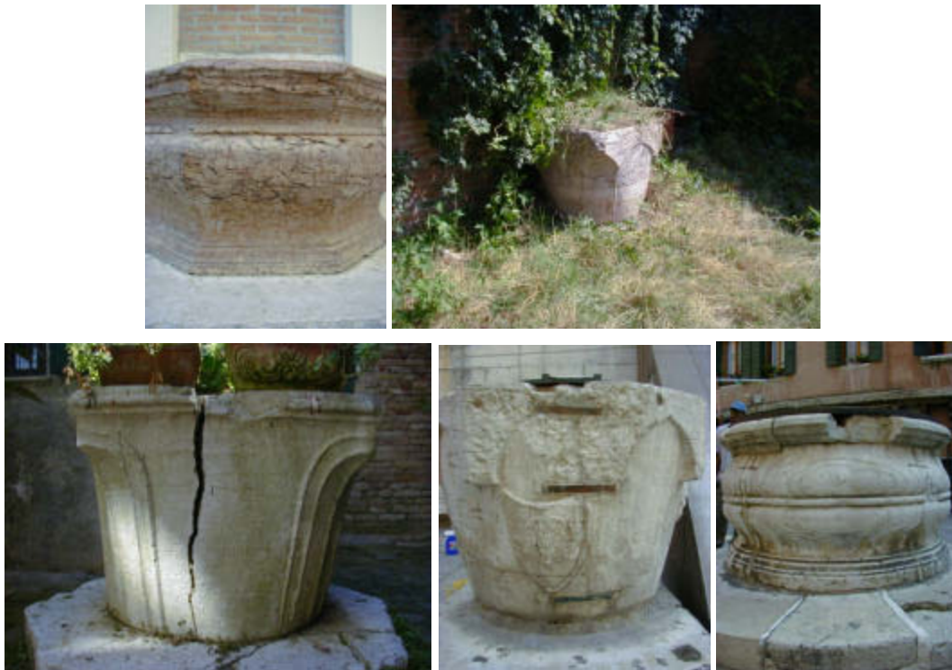
Figure 6-4 Five worst wellheads in prioritization list
