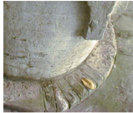
Figure 5-8 Istria Platform Repaired With Brick
