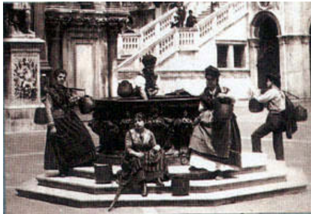
Figure 3-1 Activities Around a Wellhead
