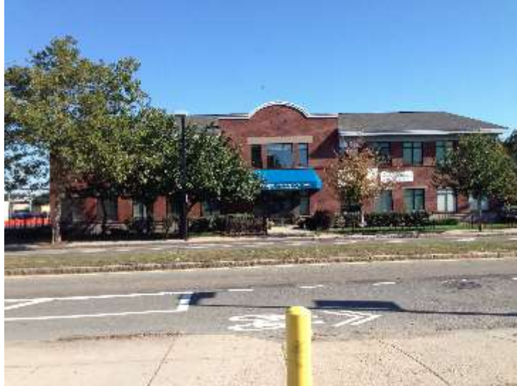
Figure 16: Vulnerable features at the First Community Health Center (original photo)
