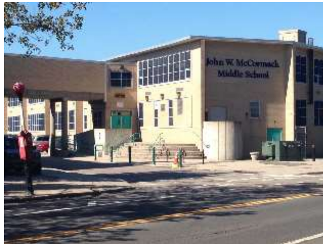
Figure 18: The John W. McCormack School with raised doorways and windows (original photo)
