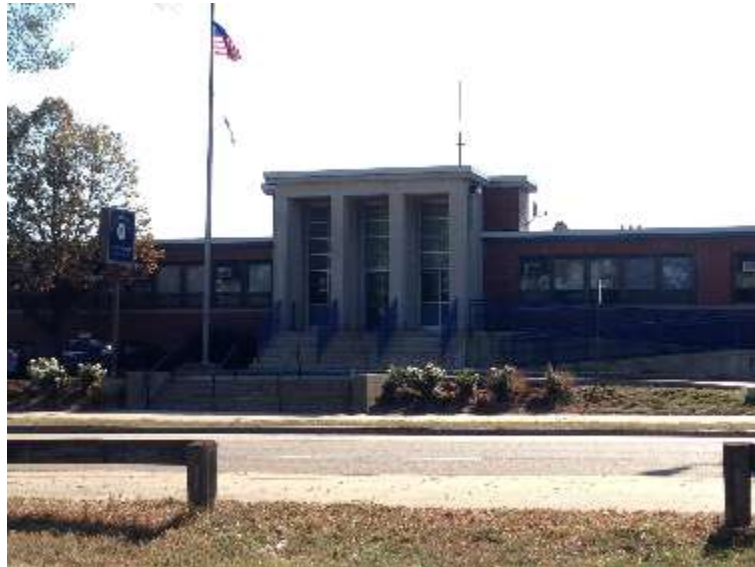
Figure 12: State Police Station of Dorchester, MA has raised doorways and windows (original photo)
