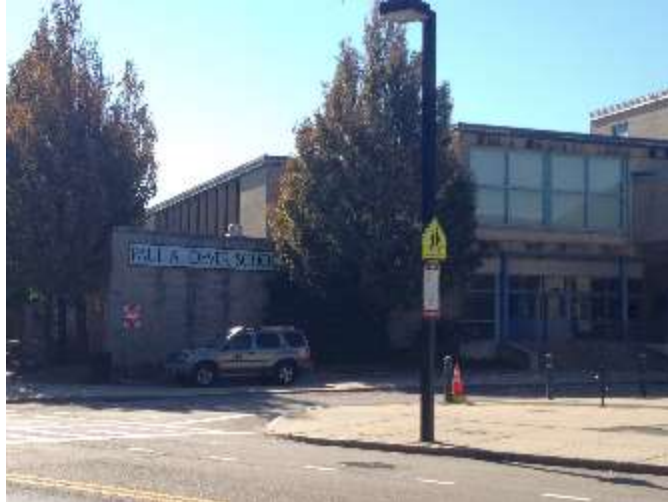
Figure 19: Paul A. Dever Elementary School in Columbia Point (original photo)
