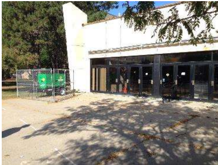
Figure 15: Ground level doors at the Bayside Expo Center (Original Photo)
