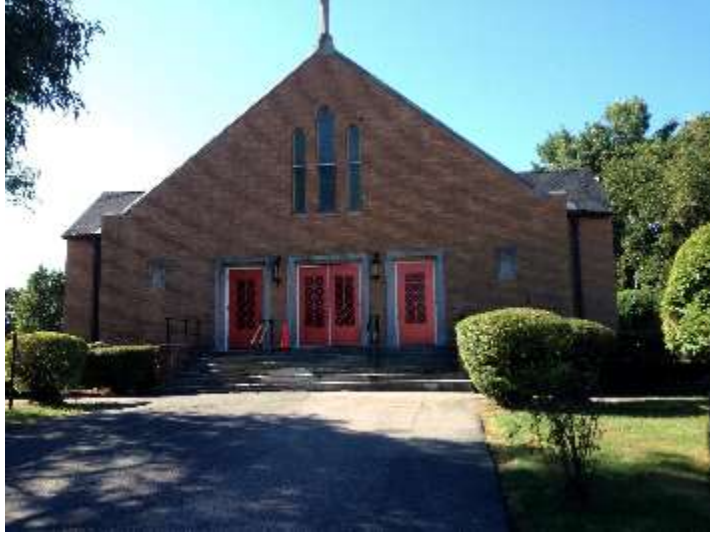
Figure 23: St. Christopher's Church (original photo)
