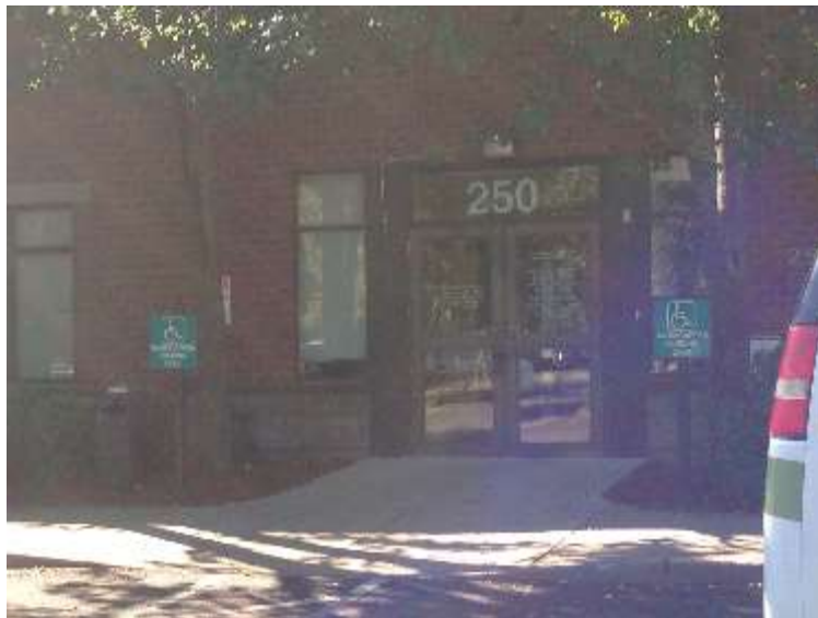
Figure 17: Ground level doorways on the Harbor Point Luxury Apartments (original photo)
