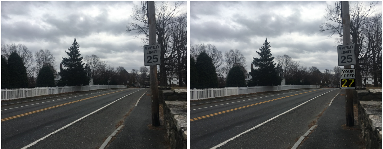
Figure 26: Before installation (left) and after installation of Radar Speed Feedback Sign
