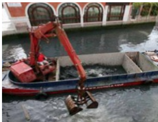
Figure 16. Deep-water dredging in a canal
